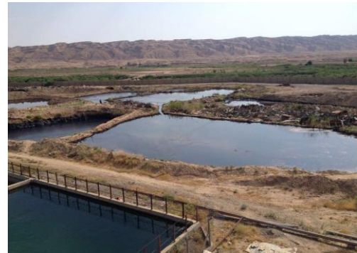
Figure (1): Ground reserve pool at Baiji gas power station
