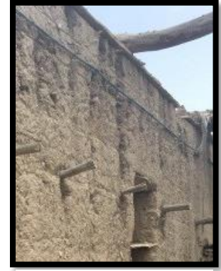
Figure 1. 14 Wall extended into Parapets
