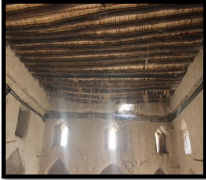
Figure 1. 15 Details of Ceiling from inside
