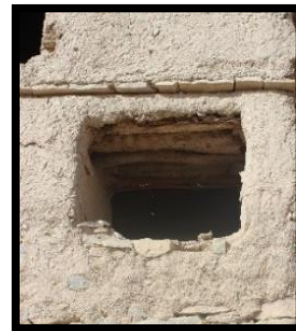
Figure 1. 19 opening in walls
