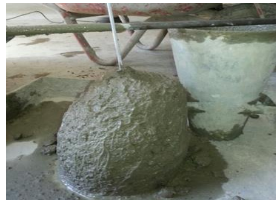
Fig -5 Slump test for Conventional Concrete
