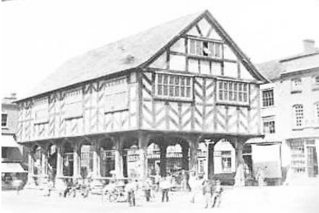
Figure 5: A typical two-storey medieval market hall with open ground floor trading, 16 th century. (Source: http://www.victoriacountyhistory.ac.uk/explore/themes/trade-and-commerce/markets-and-fairs )
