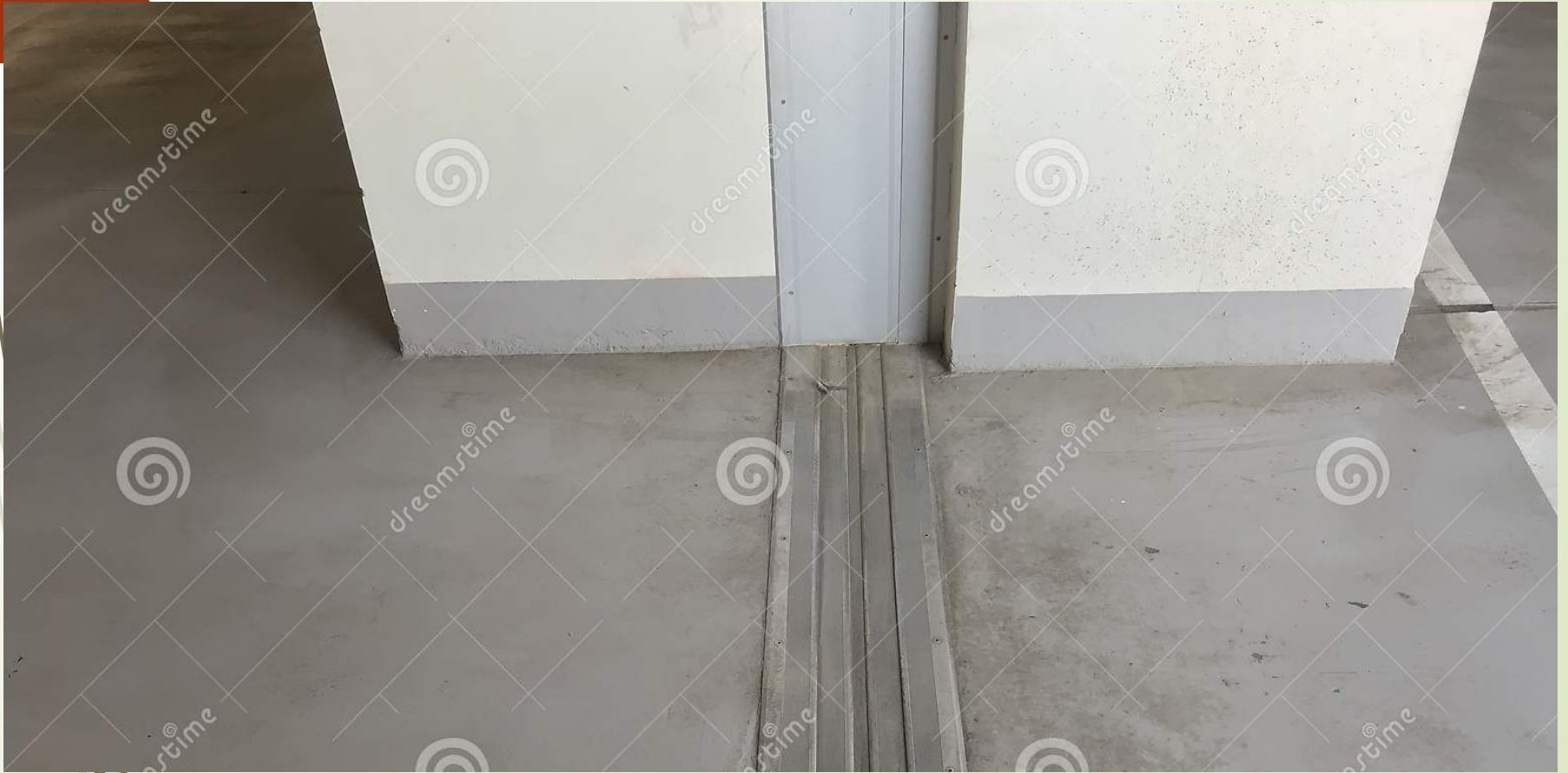
Movement Joints in Concrete Slabs
